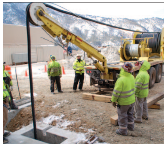
970' vertical single-messenger MPF borehole installation.
