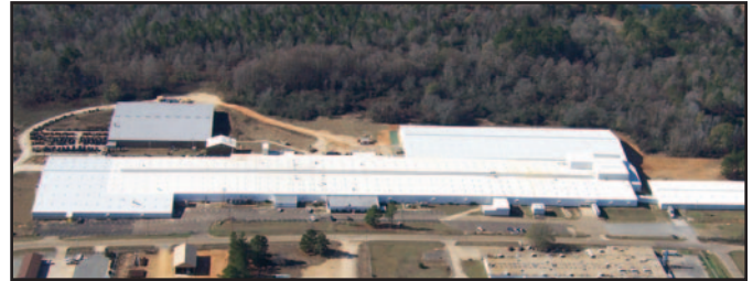
Nexans AmerCable's 400,000 sq. ft. manufacturing facility and corporate headquarters in El Dorado, Arkansas.
